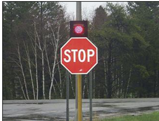
NS09- Install Flashing Beacons as advance warning (N.S.I)
