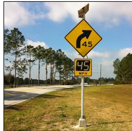
R26- Install dynamic/variable speed warning signs
