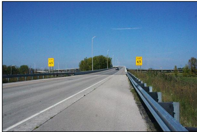
R21- Improve pavement friction (High Friction Surface Treatment)
