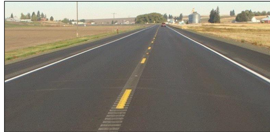
R30- Install centerline rumble strips/strips
