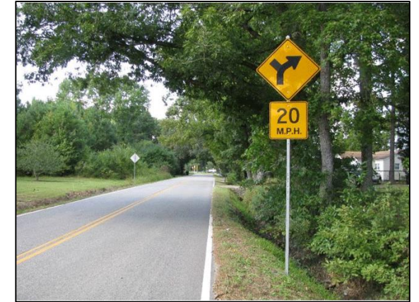
R24- Install curve advance warning signs
