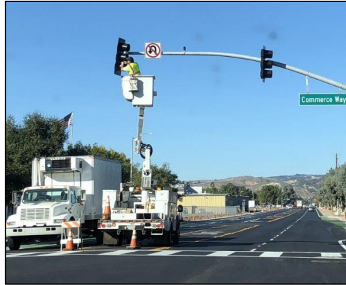
NS03- Install signals
